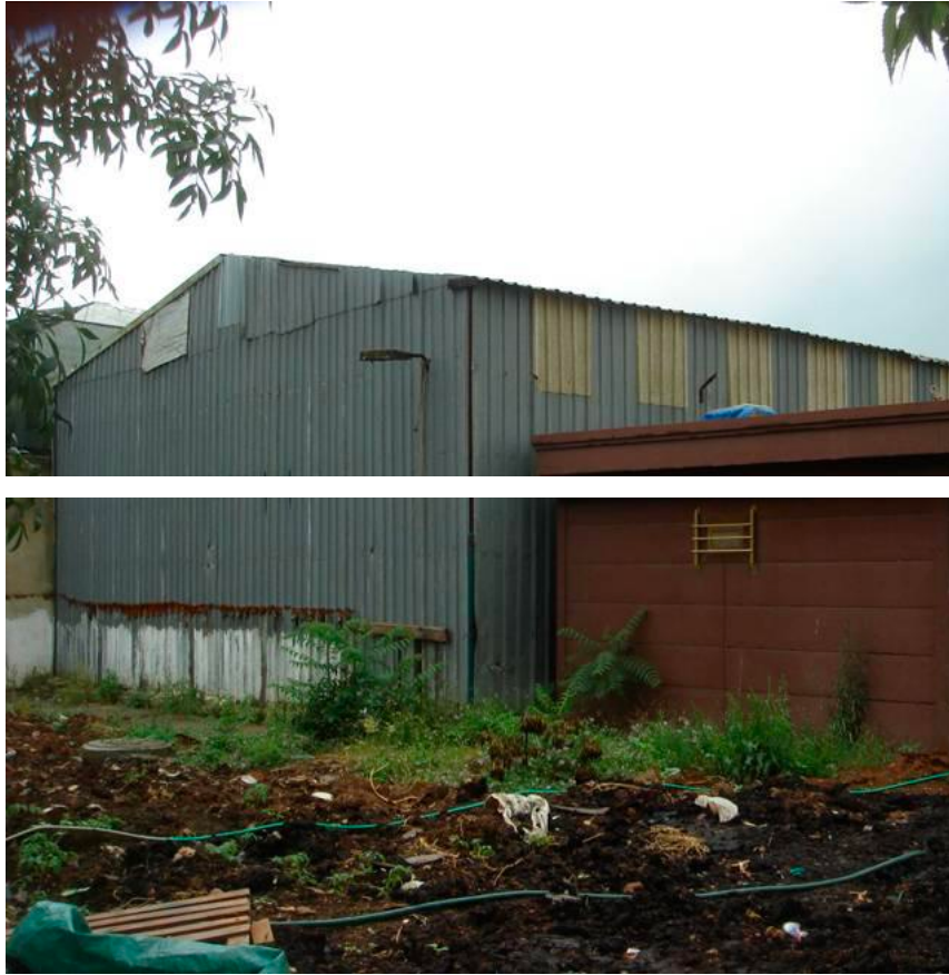
Fig.101 - Aya Nicola Shed Building used as Municipal depots before the renovation.
