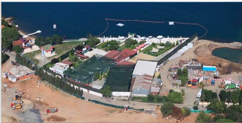
Fig. 100- Site View of Aya Nicola Shed Building used as Municipal depots Source: Islands Museum web page
