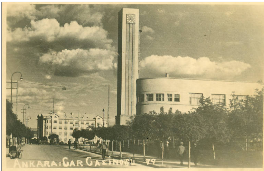
Fig.120- Ankara Train Station Club Building and Clock Tower
