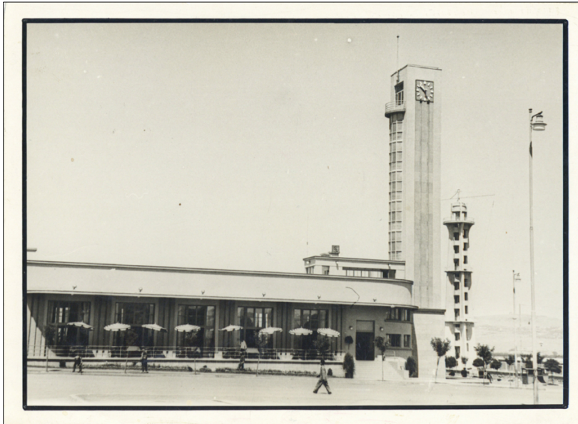
Fig. 130- Train Station Club Building Source: Salt Research Archive 445
