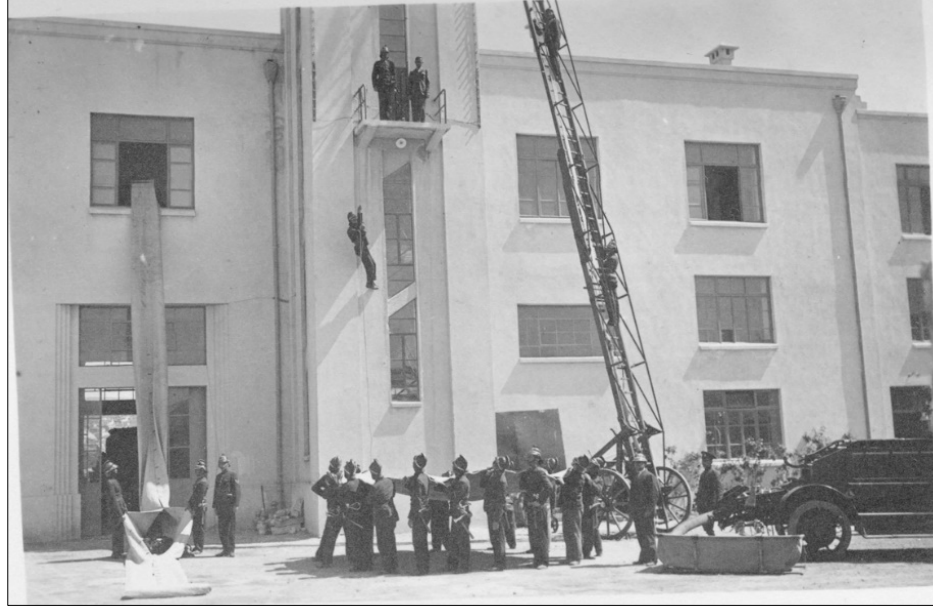
Fig.74- İzmir Fire Station Building, rear facade
