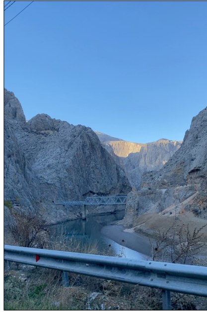
Fig. 19- Şırzı Bridge, 2023 Photo: by the Author
